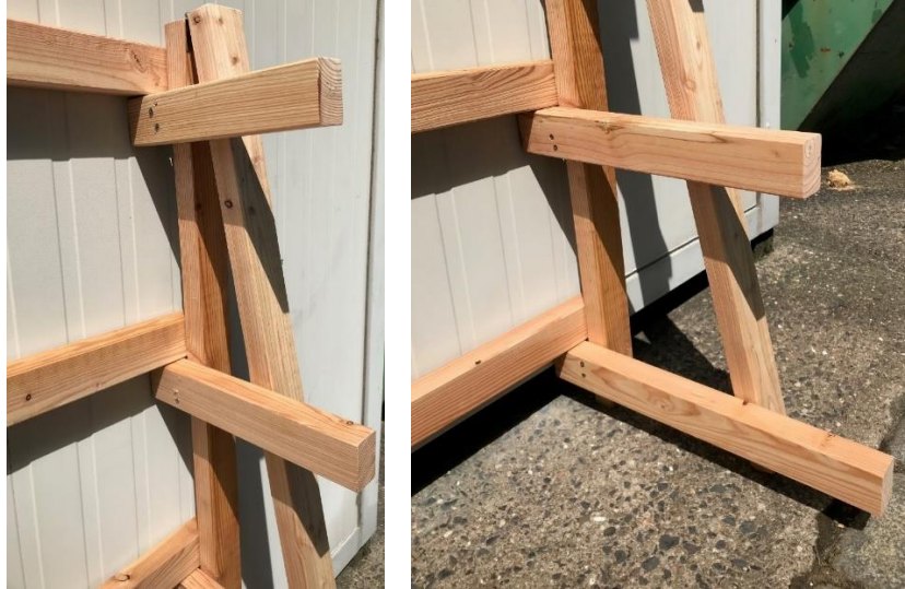
Figure 16: Assembling of the struts – in detail.
