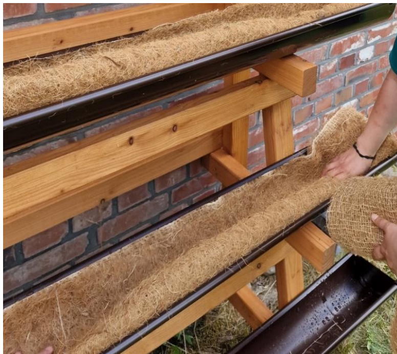
Figure 26: Placing the coconut fiber mats in the gutters.
