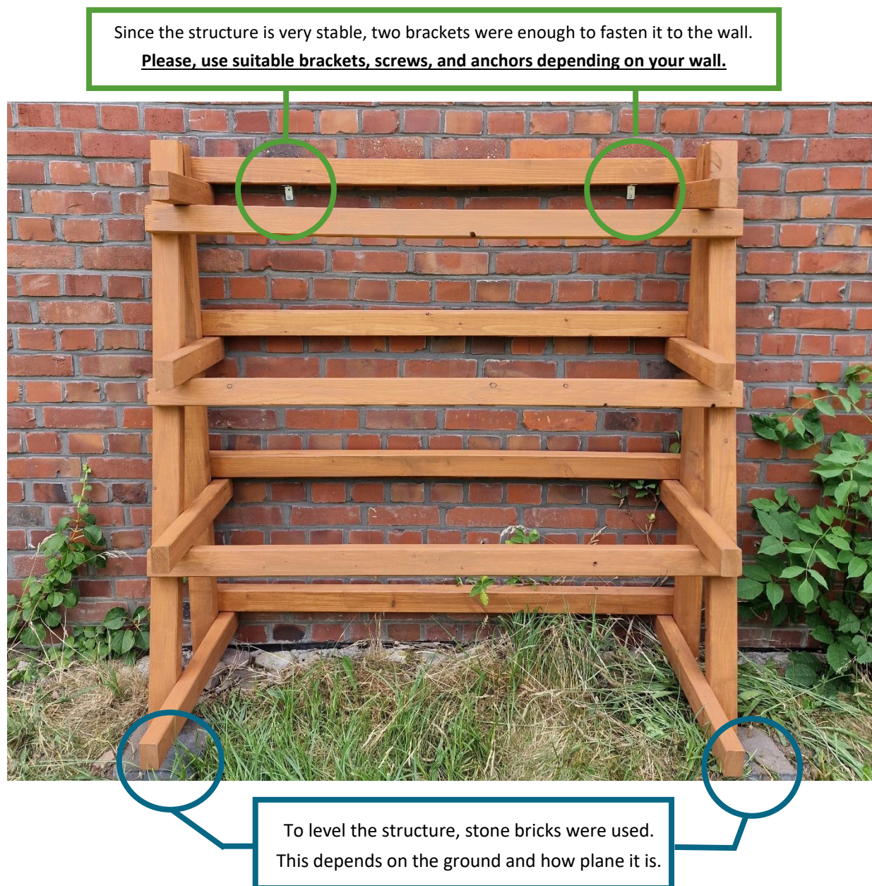
Figure 19: Placement of the frame in its final position.
