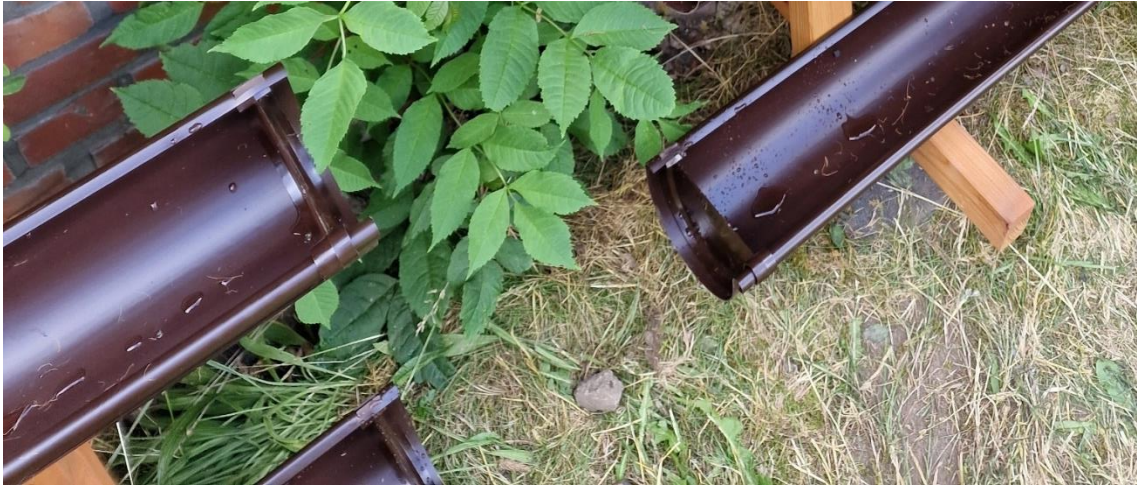
Figure 22: Rain gutters fastened to the frame.
