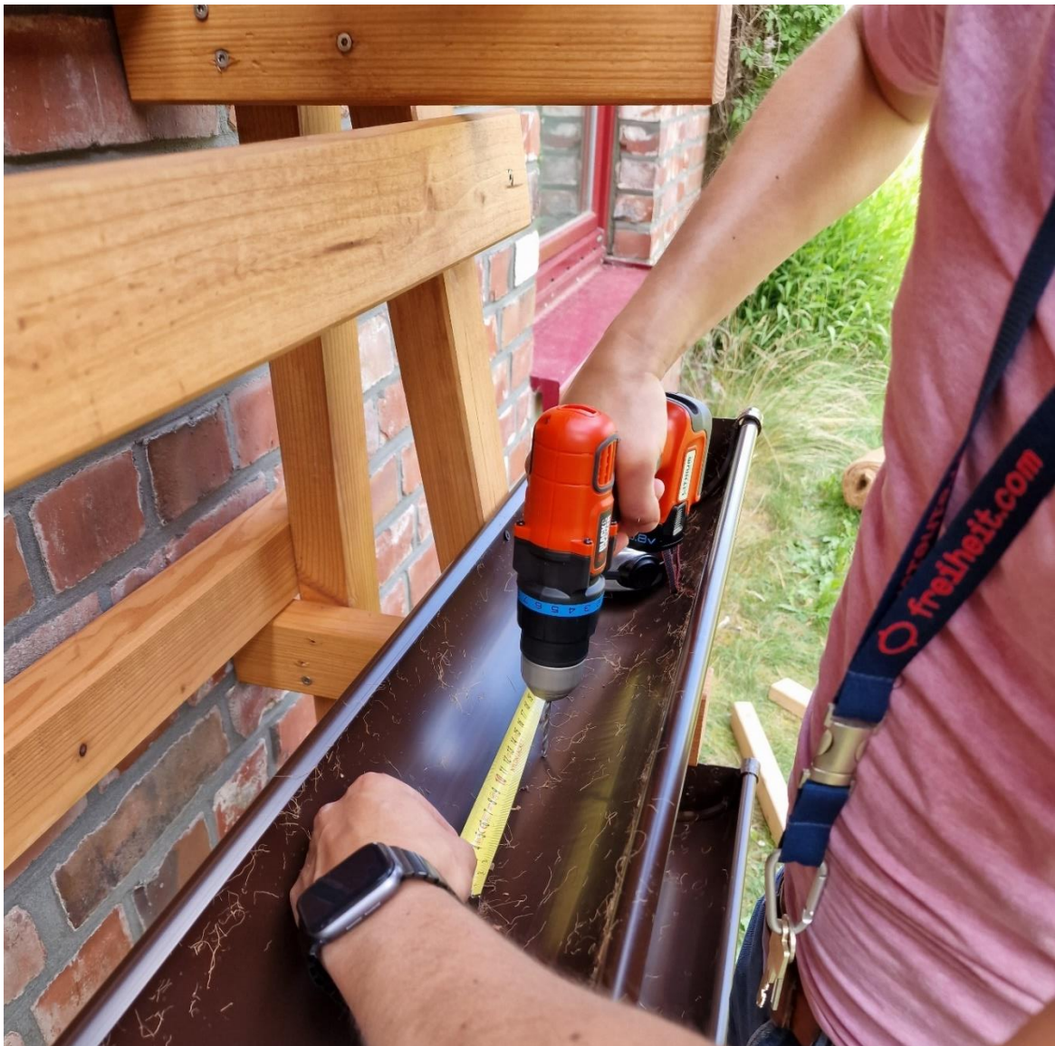
Figure 24: Drilling the drainage holes.
